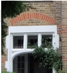
Rubbed brick flat arches in gable and over door – Inglis Road
