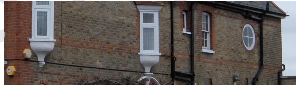
London stock brick used on the sides of houses with string courses of red brick
