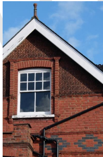
London stock brick used on the sides of houses with string courses of red brick
