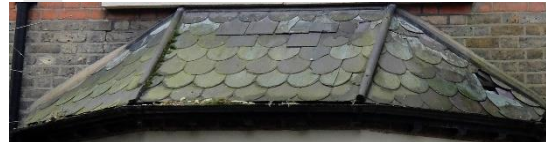
Fish tail slate tiles on dormer - Freeland Road and on turret roof & canted bay - Inglis Road
