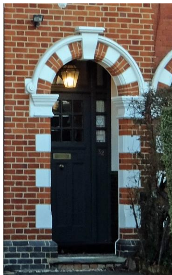
Arched brick recessed door surround such as on the West side of Western Gardens, Twyford Avenue, and on the corner houses where entrances are on the sides. These tend to have glazed tiles on the lower section of the recess.
