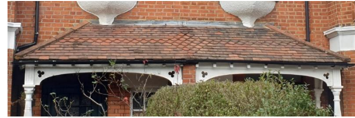
Tiling detail is continuous across porch roofs between pairs of semis - Layer Gardens
