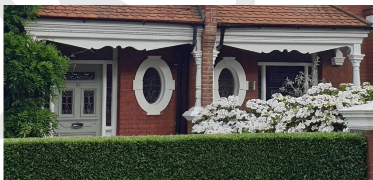
Arched brick recessed door surround such as on the West side of Western Gardens, Twyford Avenue, and on the corner houses where entrances are on the sides. These tend to have glazed tiles on the lower section of the recess.
