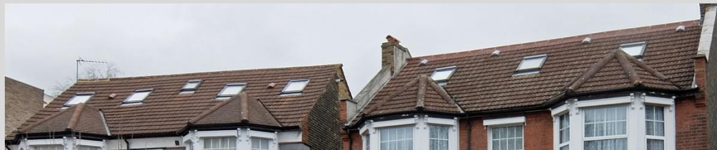
Concrete tiled roofs and too many and unaligned dormers detract from the front of the house
