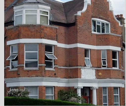
Wrong fenestration, top hung rather than sash windows and made of uPVC.
