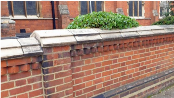
St Martin's Church wall detail showing fireclay coping on walls and pillars and the wall stepping down in height due to slope in Hale Gardens.
