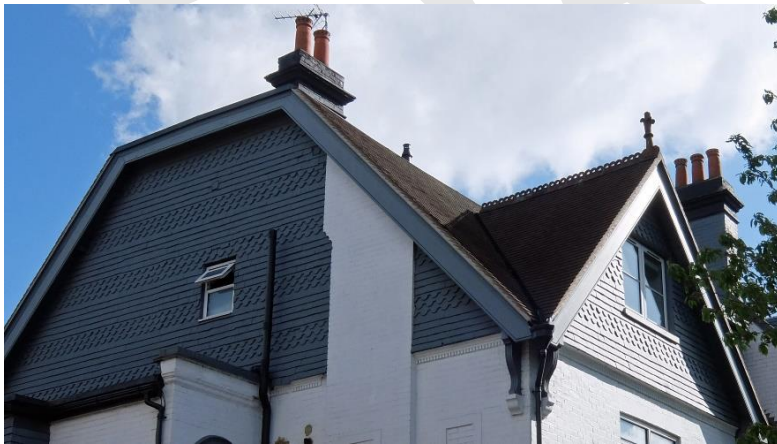
Tile hanging example, although over painted – Creffield Road
