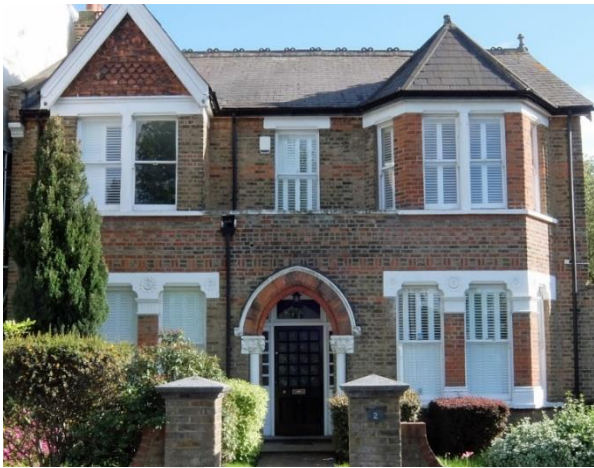
Mixed stocks and stone detailing on lintels – Inglis Road
