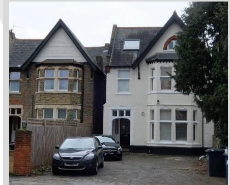
Over painting and rendering of brickwork compared to original
