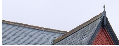
Slate roofs, and coggled crest ridge tiles and chimney detail – Creffield Road
