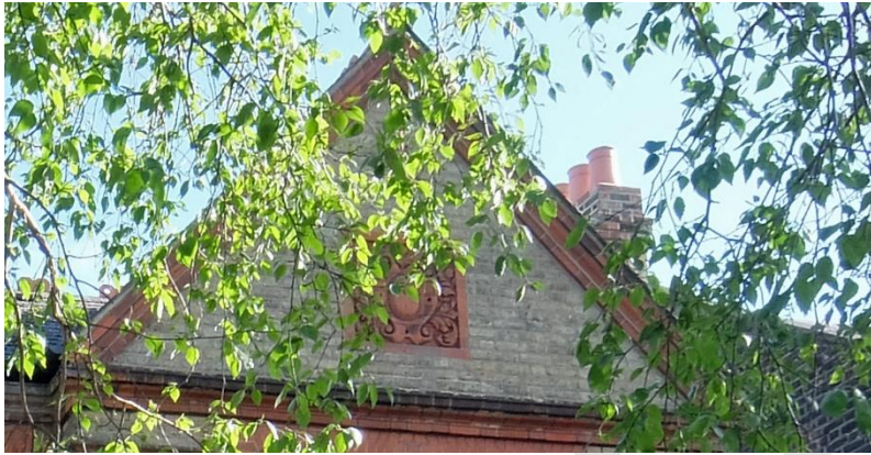
Brick and pressed clay tile inset – Inglis Road
