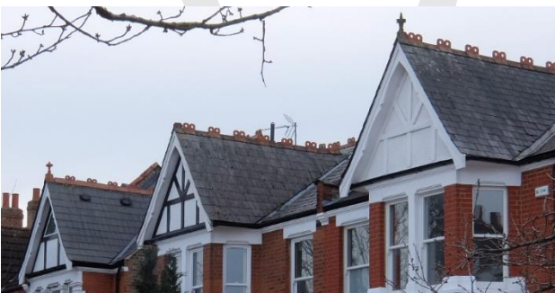
Clay and slate tiled roofs with two hole clay ridge tiles
