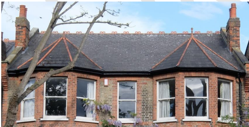
Clay and slate roofs with hit and miss two holed clay ridge tiles
