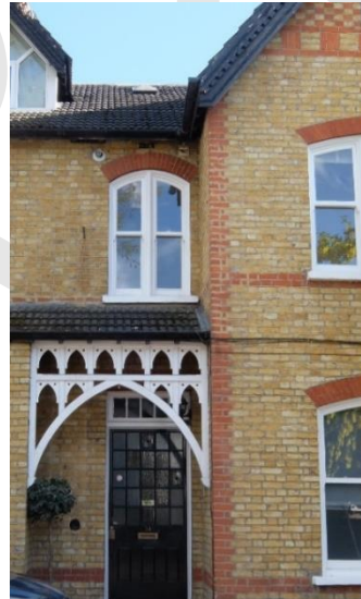
Rubbed brick flat arches over windows – Freeland Road
