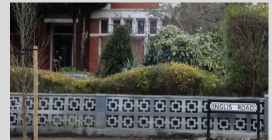
Inappropriate materials for wall that don't match surrounding brickwork
