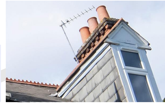
Slate roofs, and coggled crest ridge tiles and chimney detail – Creffield Road
