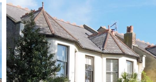
Fish tail slate tiles on dormer - Freeland Road and on turret roof & canted bay - Inglis Road
