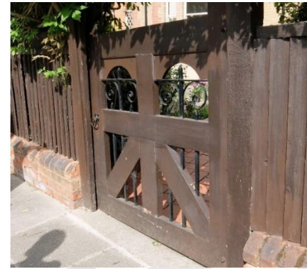
Rare instances left of low brick walls, with closeboard fence and timber gates - Inglis Road
