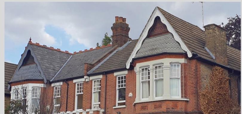
Concrete tiles rather than slate detract from the roof scape
