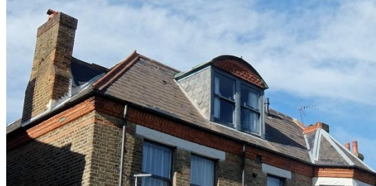
Slate roofs, and coggled crest ridge tiles and chimney detail – Creffield Road
